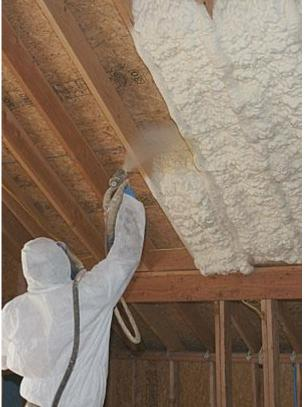
Made from polyurethane, this product reduces air leakage better than any other type of insulation. It fills the nooks and crannies of unusually shaped building cavities easily.
